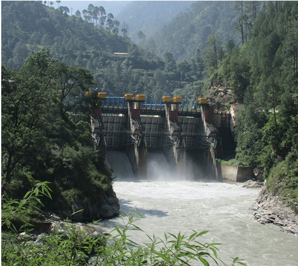
Maneri Bhalu dam, Uttarkashi district, Uttarakhand, India (photo by the author)
