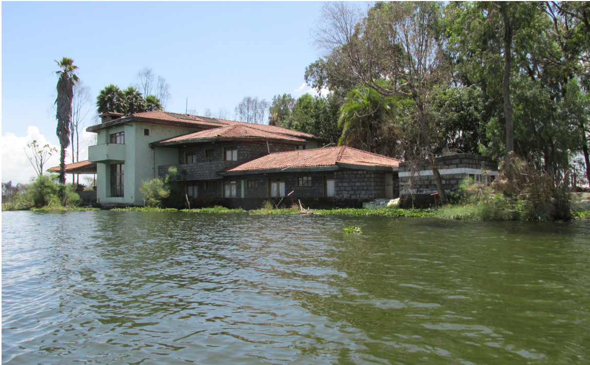
The abandoned house of the former owner of a flower farm that got into financial trouble. The house was constructed at a time when lake levels were lower.
